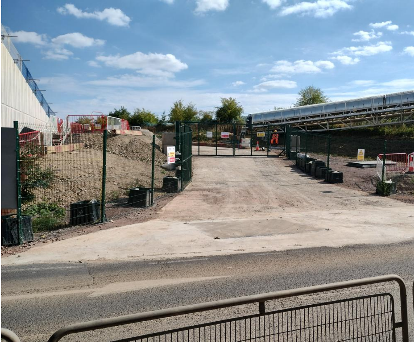
Installation of Sheet Piles for Copthall Rail Siding – 14/07 to 20/09
