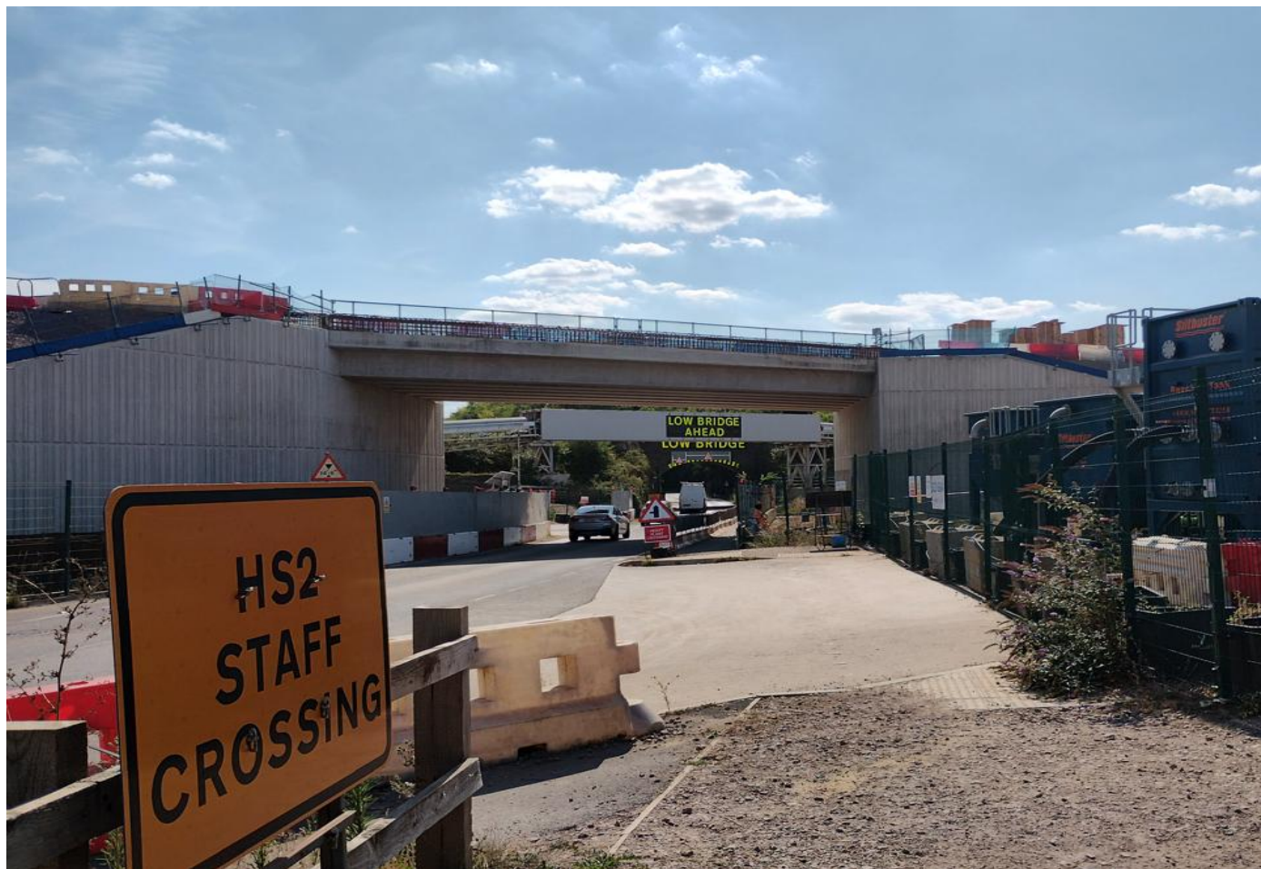
Photo shows the Eastern side of the Haul Road Crossing which remains open for HS2 traffic exiting from Site Access on the southern carriageway near the new HS2 Overbridge
